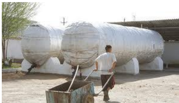
Large insulated biogas digesters in Uzbekistan made from old train cisterns.
