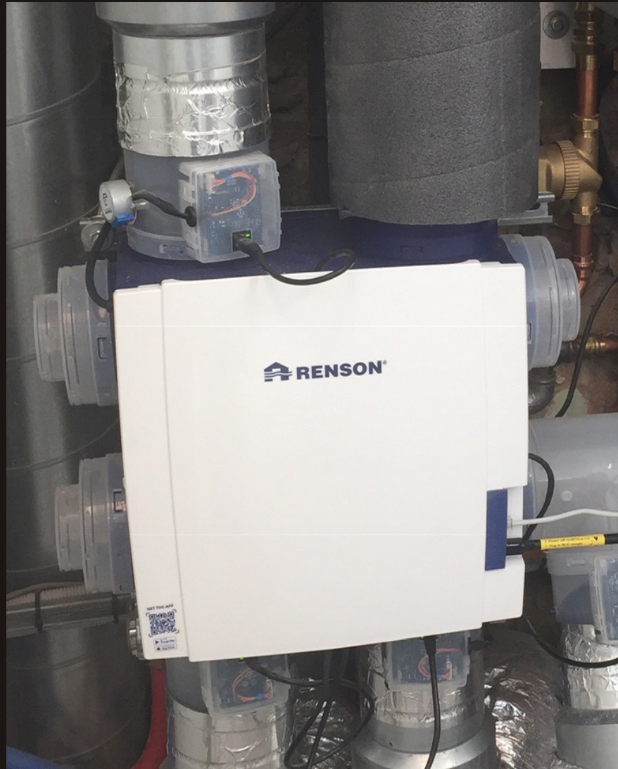
Renson's smart, sensor-controlled Health Box 3.0 ventilation system
