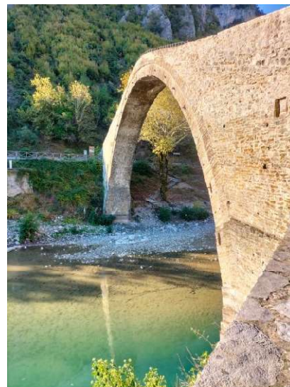
8 The bridge of Konitsa
