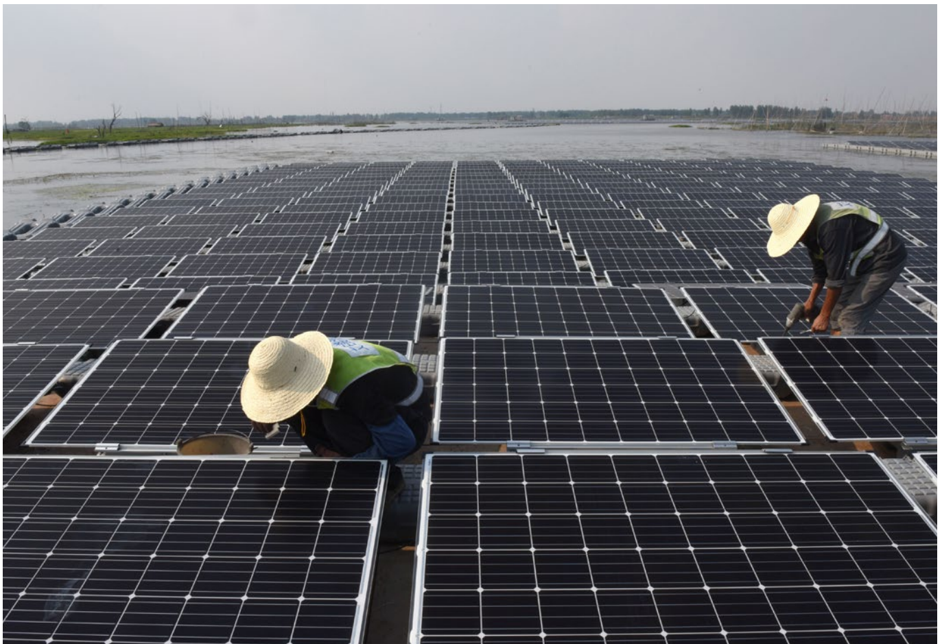
Chinese workers install panels at the Huainan solar farm in Anhui province. Constructed on the site of a former coal mine and comprising over 160,000 solar modules, the array is one of the world's largest floating photovoltaic solar plants and has capacity to power more than 15,000 homes (2017).
